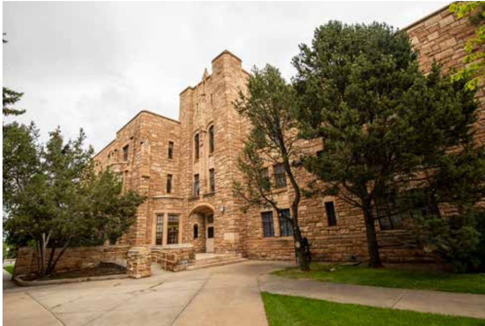
McWhinnie Hall architectural details
