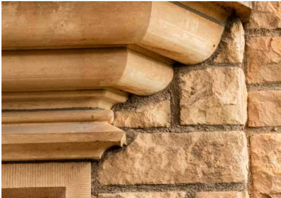
McWhinnie Hall architectural details
