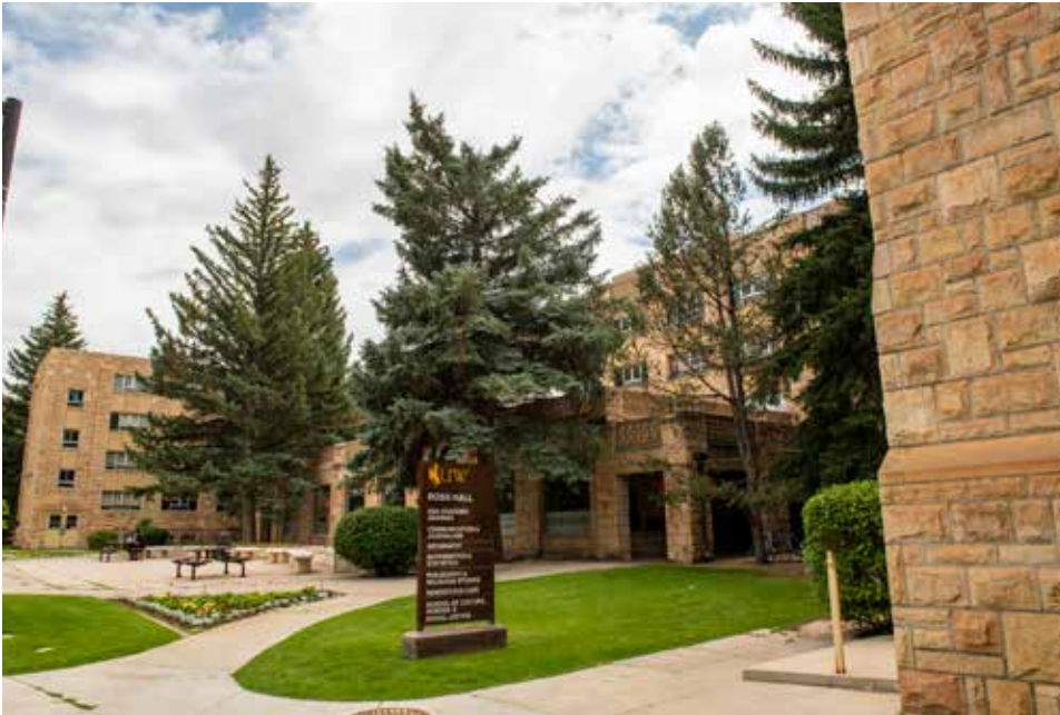
Ross Hall architectural details
