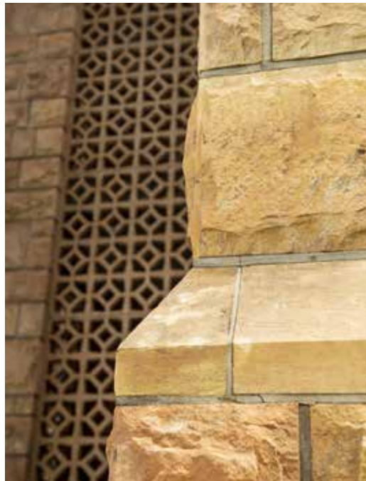
Ross Hall architectural details
